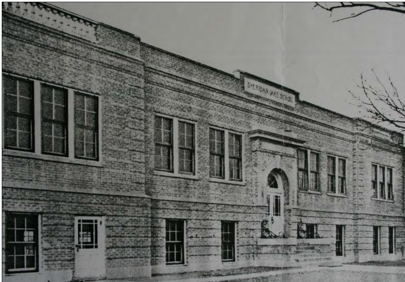
Figure 1. In this undated but apparently early view, the Sheridan Lake School displays its original windows, doors, roof balustrades, and wrought iron scrolls flanking the entrance (view east-northeast). Courtesy of Kiowa Albright Memorial Center, Sheridan Lake, Colorado.
