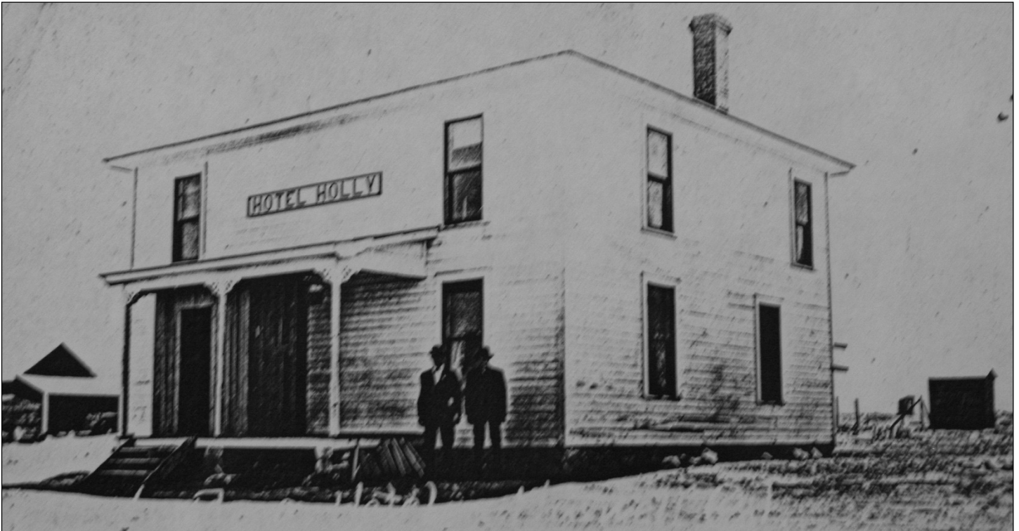
Figure 2. This ca. 1908-09 photograph (view southeast) shows the front and west wall of the Hotel Holly, with its original horizontal clapboard walls. Courtesy Haswell Community Center, historic photograph display.
