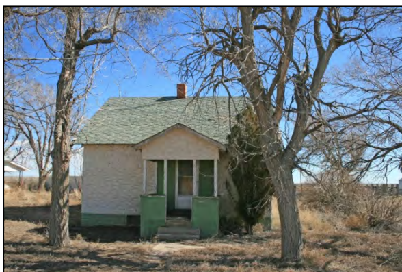
View east of the Andy Reinert house, 2012
